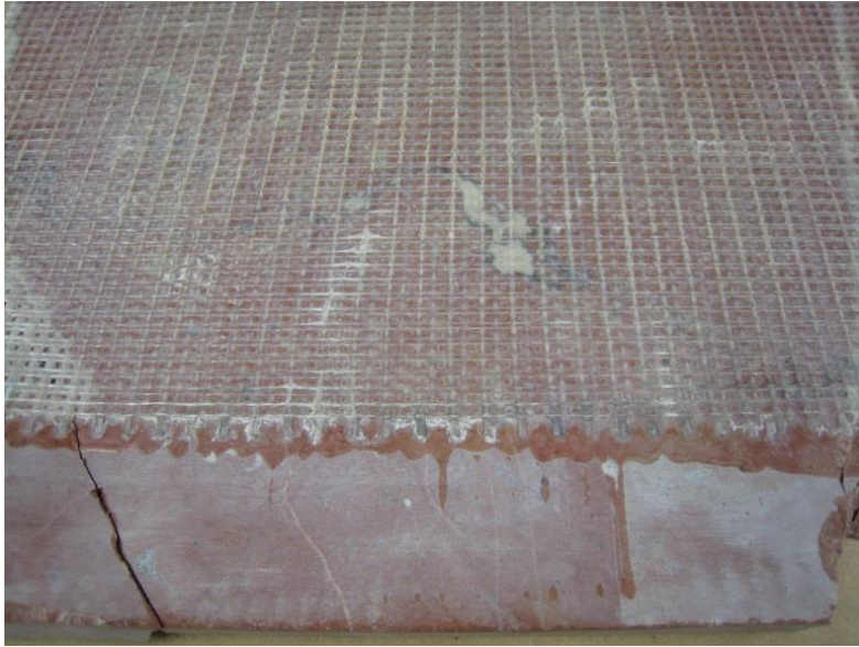
This example shows a double layer of reinforcing mesh, and the tile is still cracked.
