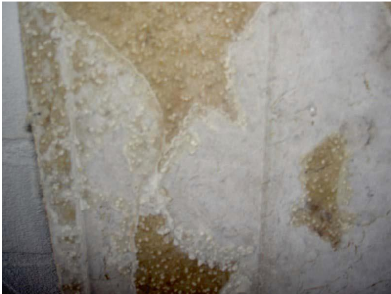
This polyester resin-backed tile was installed in an external application with a cement-based adhesive. Over a two-year period, the adhesive's cement decomposed the resin, resulting in breakdown and de-bonding.
